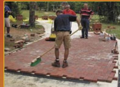
applied and the broom is constantly pushed forward (no sweeping action), it leaves the right amount of sand on top of the pavers for filling the joints. Alternatively, when more pressure is applied and a sweeping action is used, it works great for job site clean-up. The ends of the broom head are rounded to reduce splitting (square ends split easier and more often than rounded ends).
