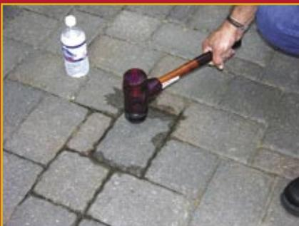
1. In the event pavers on an existing application need to be extracted, pour water around the joint. Then tap the paver to be extracted and the pavers surrounding it. This will help lubricate the joint and loosen the paver.
