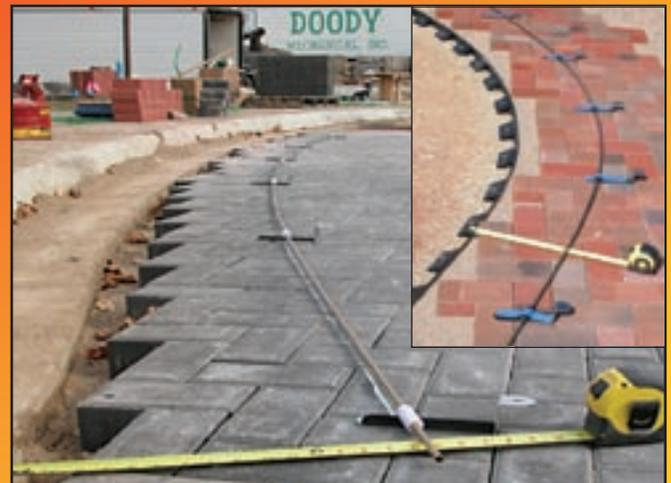
After the pavers have been marked, remove the FLEXMARKER from the pavers before cutting. **Note:** If PAVE EDGE has been installed first, follow the steps above, but measure the soldier course distance from the wall of the edging to properly align the Flex Poles for marking.
