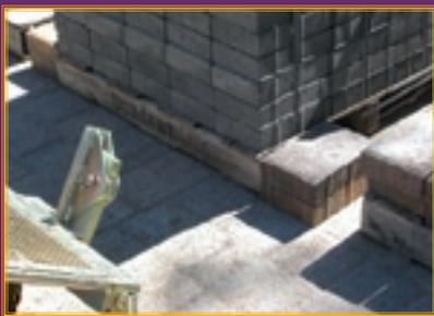
If the first Band hangs over the edge of the pallet, stack two 60 mm pavers on both sides of the pallet. When the **PAVERCART** is placed against the band, the feet will rest on top of the stacked pavers and raise the cart up.
