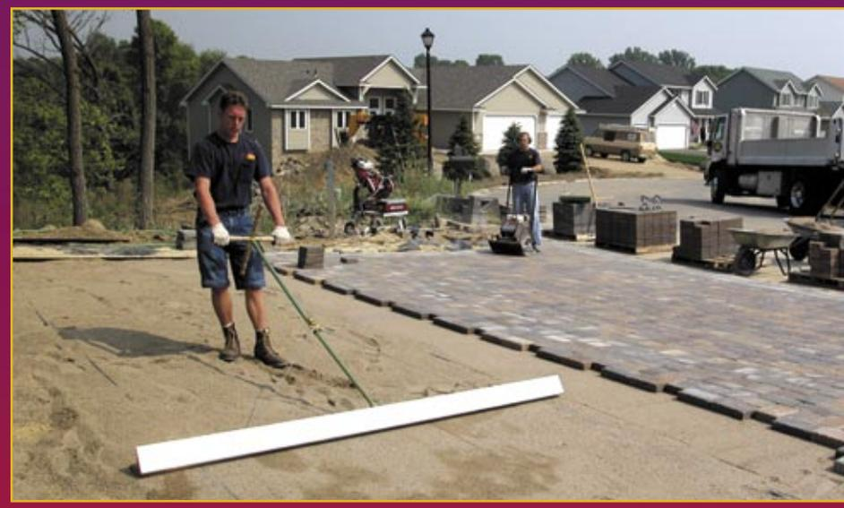
Using your existing screed rails, edge restraint, (**PAVE EDGE**) or curbing, you can screed the job faster and with more accuracy. Made of lightweight hollow core extruded aluminum the **SANDPULL PRO** will not lift off the screed rails when material is building up in front and will not sag or bend under load.
